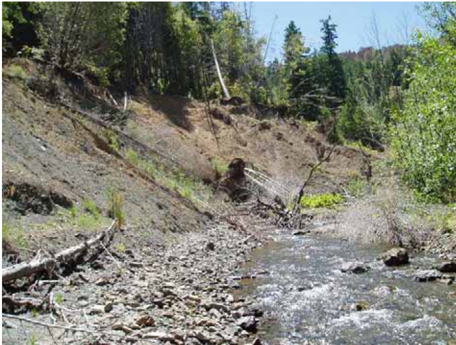
Photo 5-10. Streamside Mass Wasting along Harmonica Creek.
