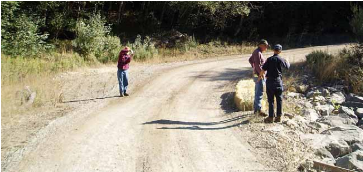
Photo 5-2. Mainline Road Approaching Bear River Bridge.
