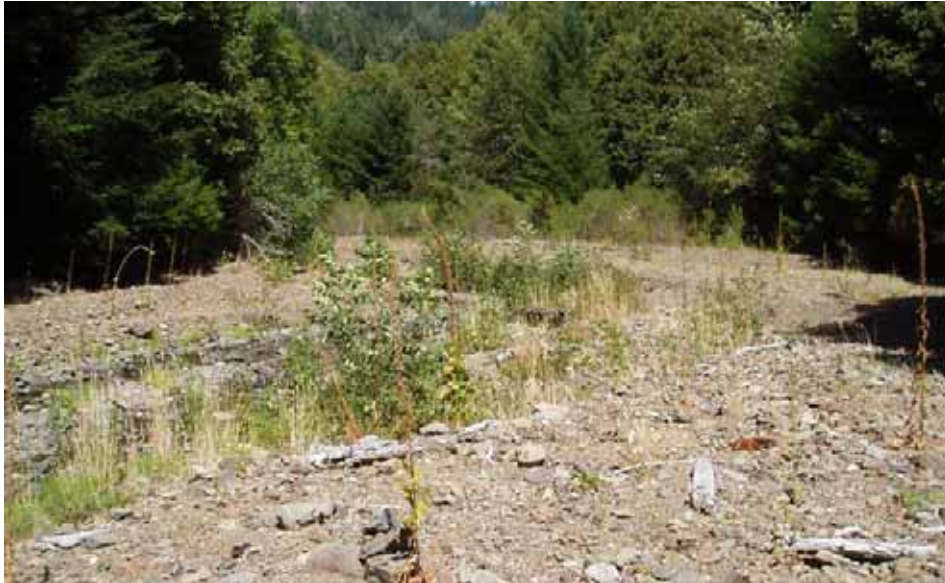
Photo 5-16. Landslide Deposition in Lower Brushy Creek.
