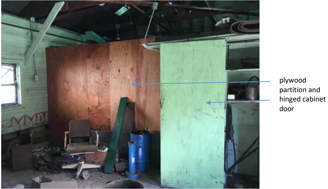
Figure 233 4.B partition across the width of room, horizontal lateral siding.
