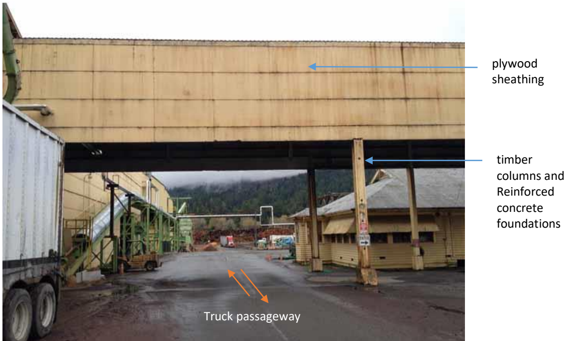
Figure 30 2.A east view of the structure
