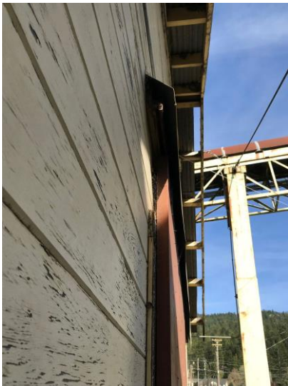
Figure 77 wood horizontal siding (typical) on exterior wall.
