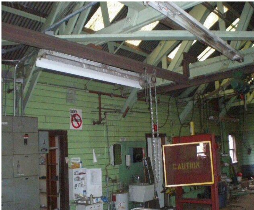
Figure 91 3.A horizontal interior siding, truss and support brackets, pulley system, sink and various movable items.
