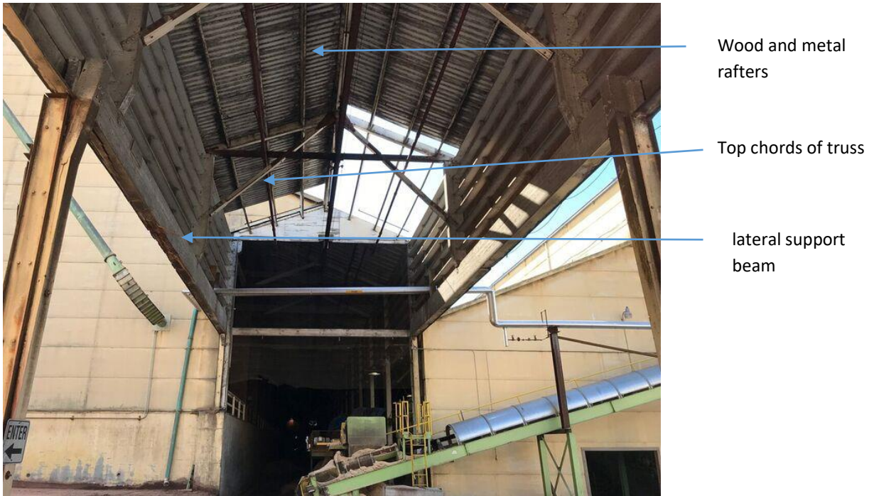
Figure 32 2.C north view of Southern Monorail Tunnel metal roof
