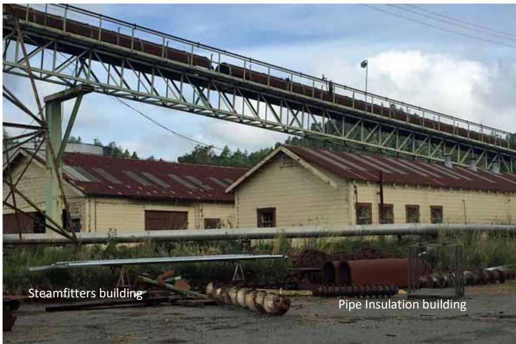
Figure 252 2.A east view of building, with double hung wood windows, frames and surrounds, horizontal wood sheathing, exposed rafters and corner boards.
