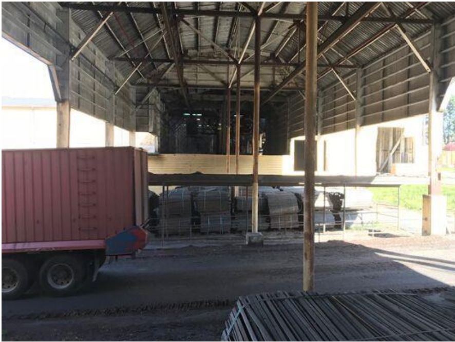
Figure 22 1F north view open ceiling and exposed truss, beams and rafters
