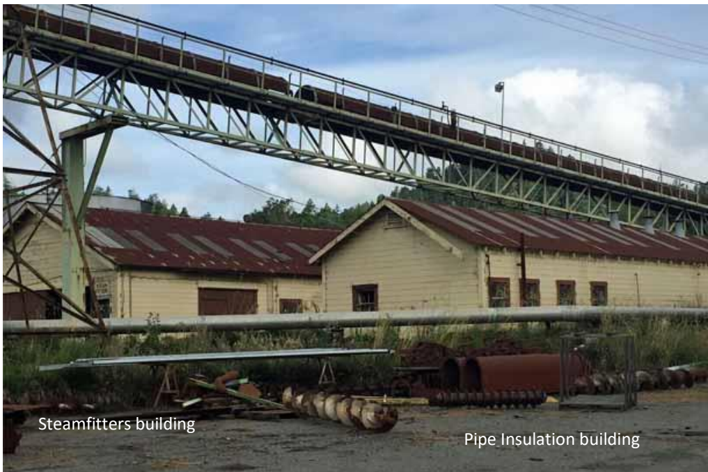
Figure 221 2.A east view of building, with double hung wood windows, frames and surrounds, horizontal wood sheathing, exposed rafters and corner boards.
