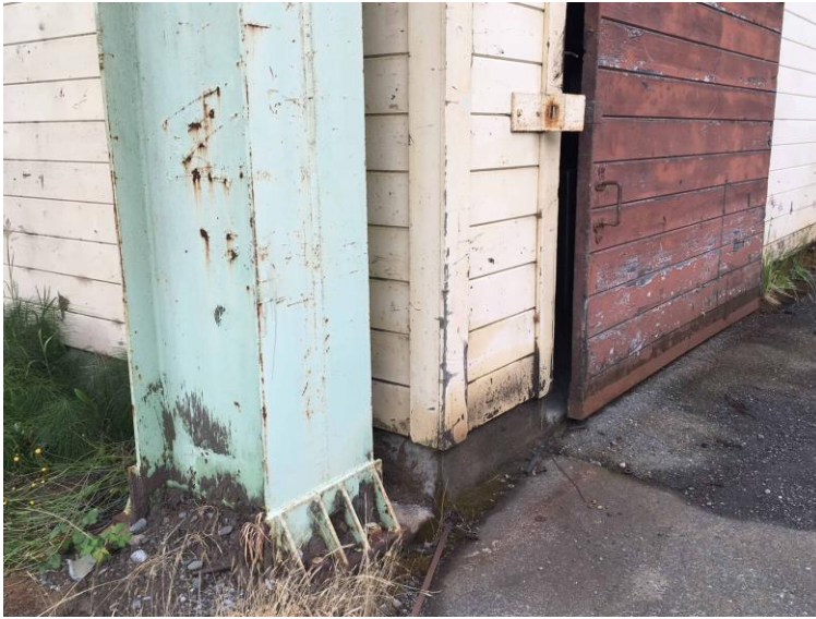
Figure 76 steel monorail column, and east elevation sliding door.
