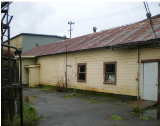
Figure 118 west side facing view with metal corrugated roofing, vents, open eaves.
