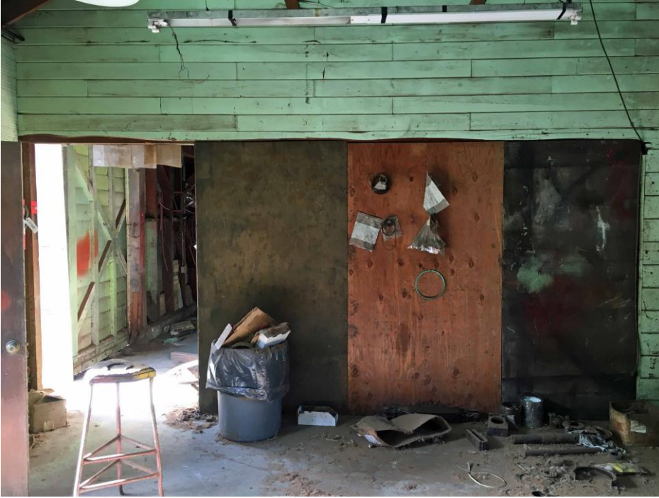
Figure 266 4.E opening and plywood boards used to reduce width of opening.
