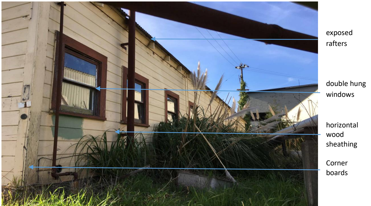
Figure 252 2.A east view of building, with double hung wood windows, frames and surrounds, horizontal wood sheathing, exposed rafters and corner boards.
