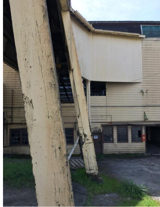
Figures 40, 41. 2.K, 2.L timber structural columns and reinforced concrete pier supports.
