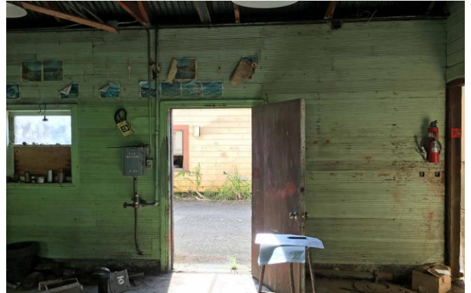
Figure 325 4.D door on the east wall to the roadway.
