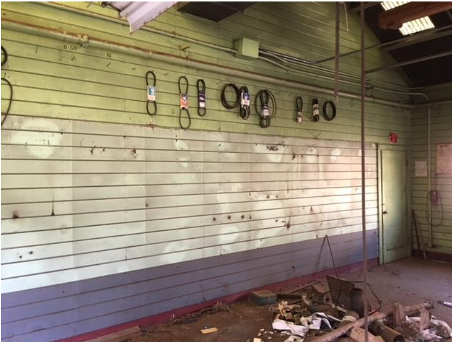
Figure 99 4.E interior partition wall running west to east, horizontal wood siding, interior door.
