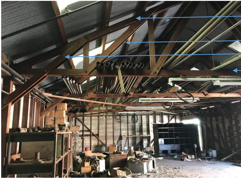
Figure 109 Steamfitters Building Truss systems
