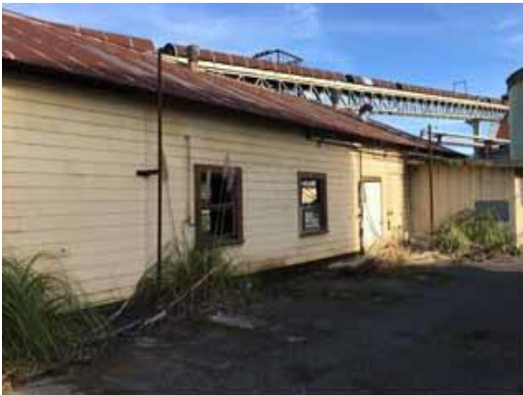
Figure 81 1.F west facing exterior wall with non-contributing addition.
