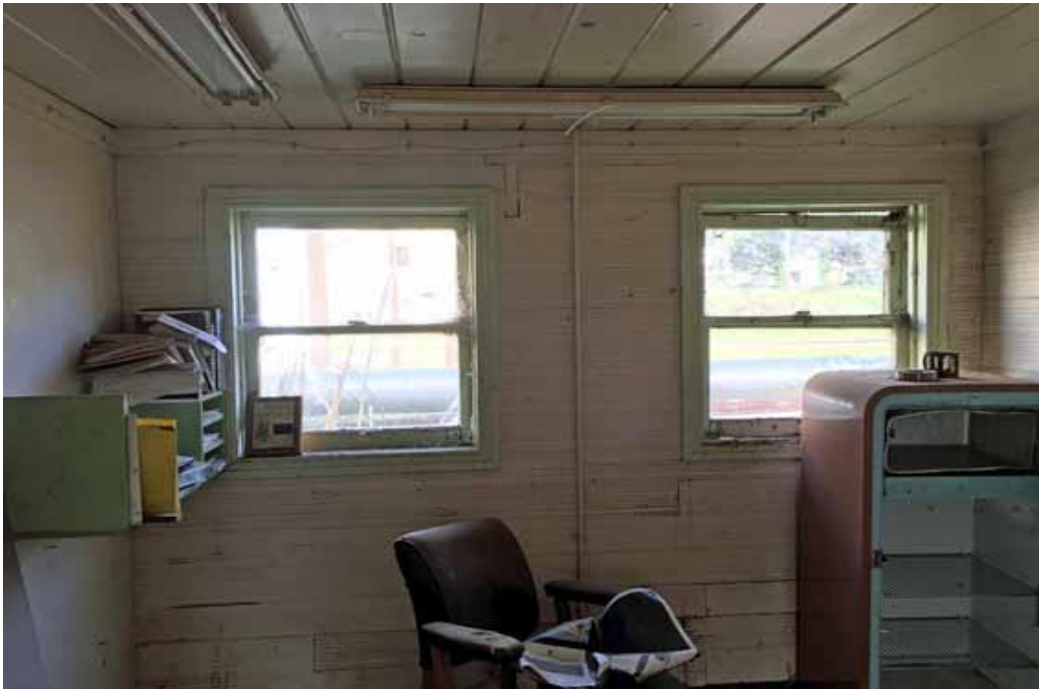
Figure 268 4.G small office space on the south side of the building.
