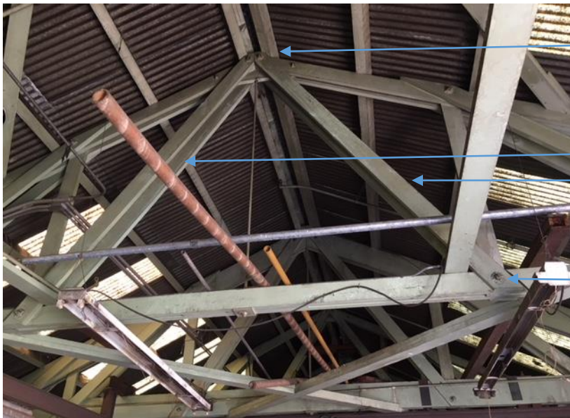
Figure 110 modified fan truss system and open ceiling.
