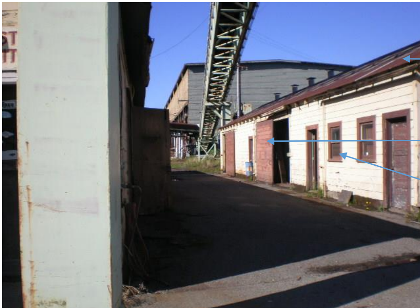
Figure 246 2.B west facing exterior under monorail line with single wood door and frames, sliding wood doors, and double-hung wood windows with surround frames. Building has open eaves, exposed rafters, and metal corrugated roofing.
