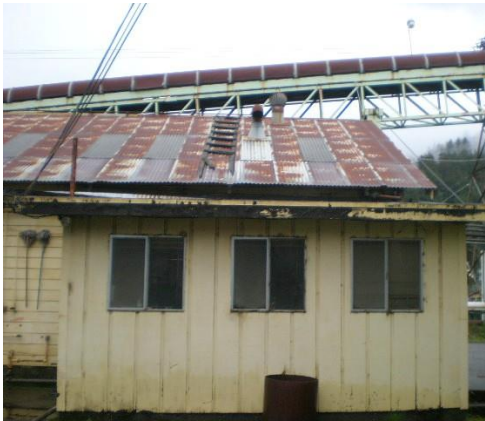
Figure 79 1.E non-contributing addition with metal corrugated roofing on original building.
