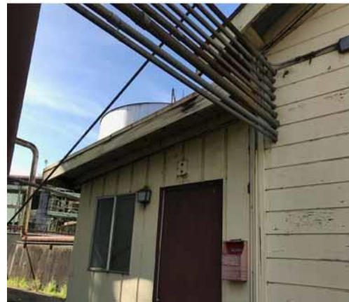
Figure 80 non-contributing addition (left) adjacent to original building with interfacing utility connections.
