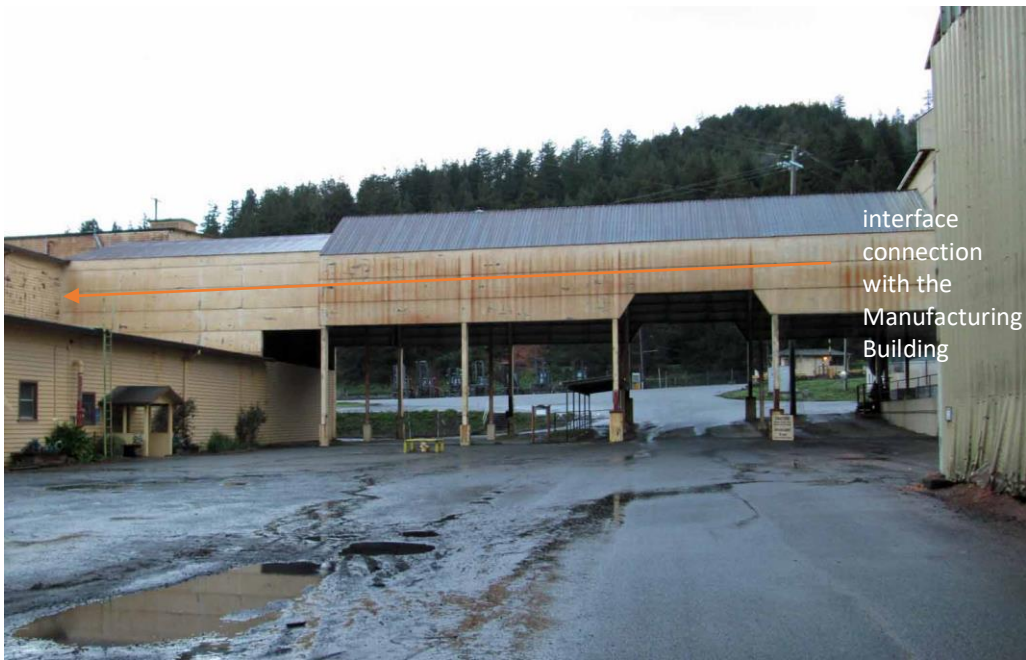
Figure 18 1.B west view of structure.
