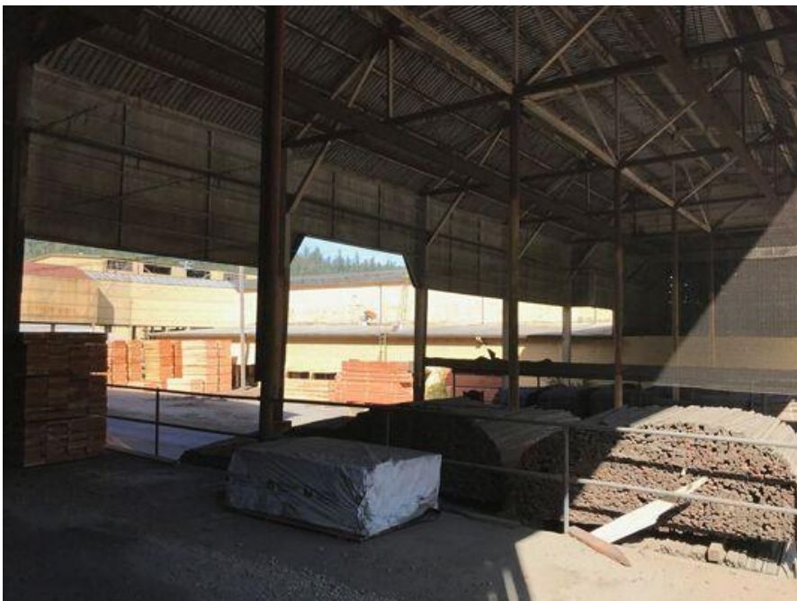
Figure 23 1.G underside of structure with exposed ceiling, wood/metal frame, and columns
