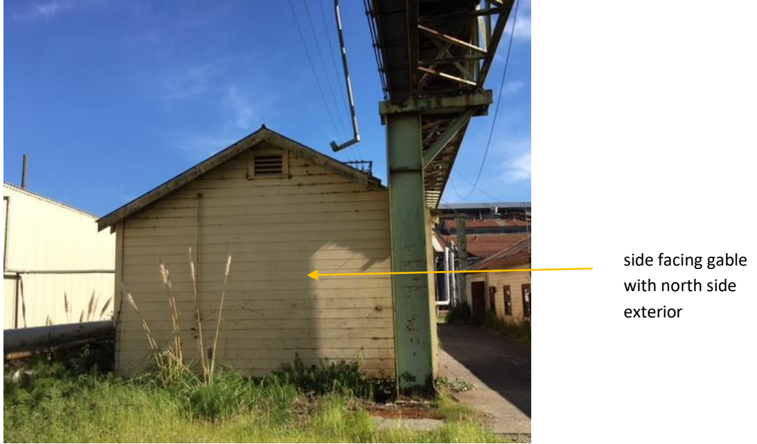
Figure 225 2.E north facing exterior wall.
