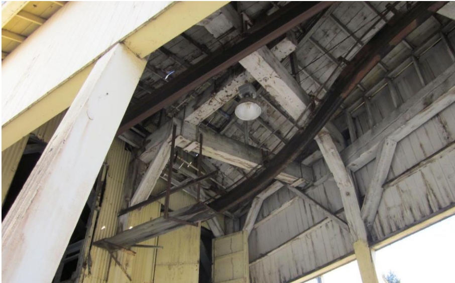
Figure 37 2.H tunnel wood frame support and curved junction of monorail track.
