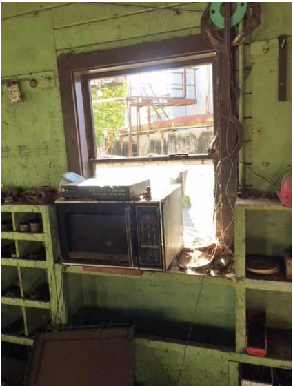
Figure 94 3.4 pair of double-hung wood windows with wood surround and frame, horizontal interior wood siding, electrical outlets.
