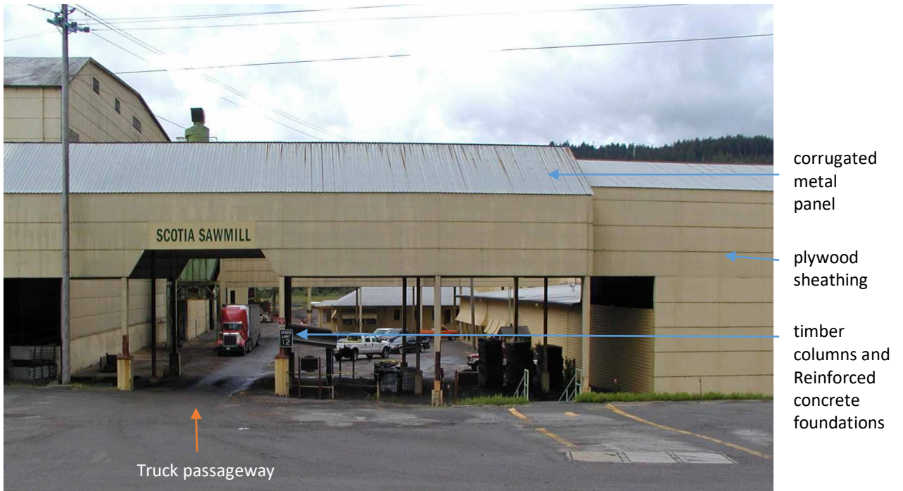
Figure 17 1.A east view of the structure.
