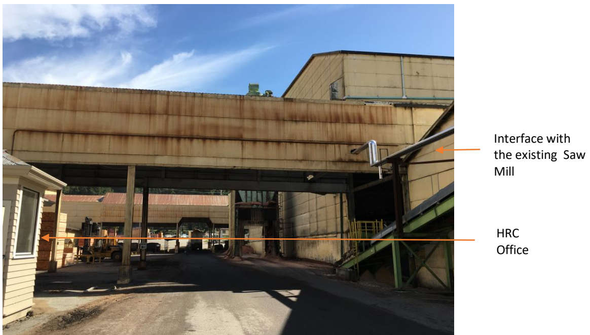
Figure 31 2.B west view of structure.
