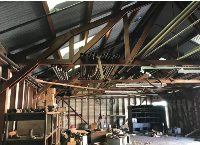
Figure 65 interior open ceiling.
