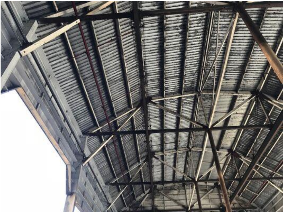
Figure 24 1.H detailed of exposed metal corrugated panel secured to wood/ metal frame.
