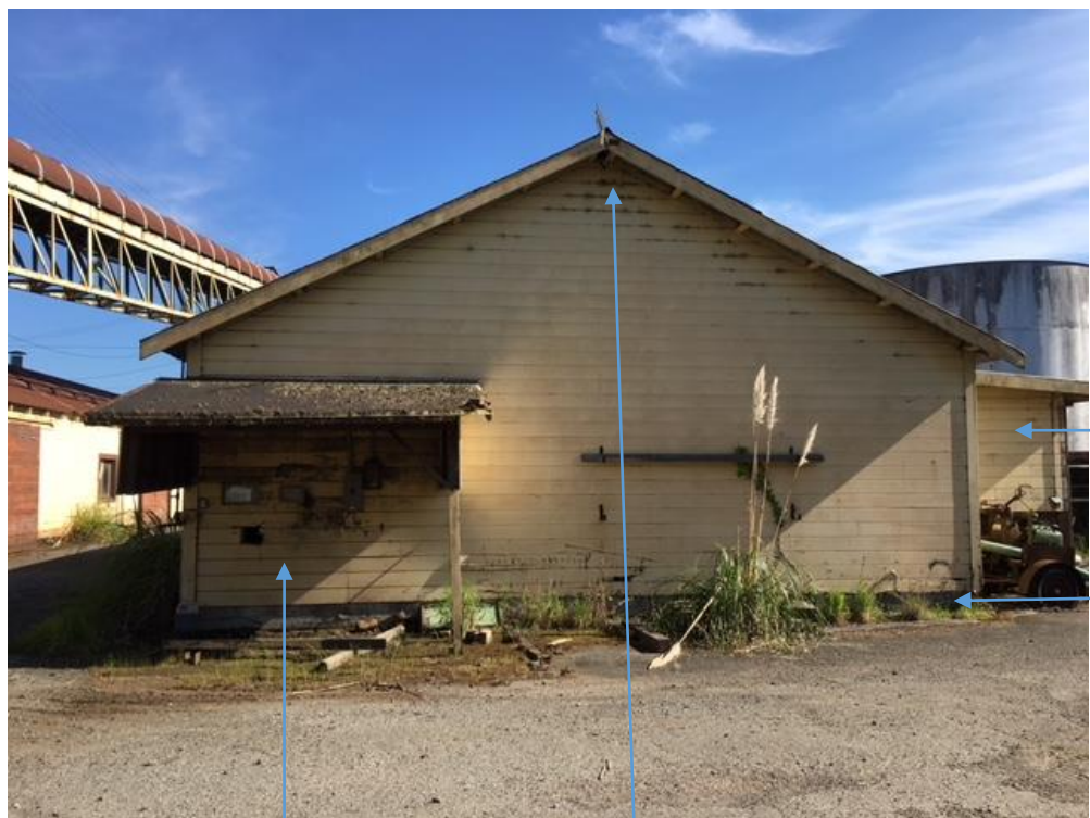
Non-contributing addition Apex of north side facing gable building, roof with open eaves and horizontal sheathing.
