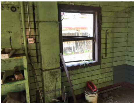
Figure 62 double hung windows.
