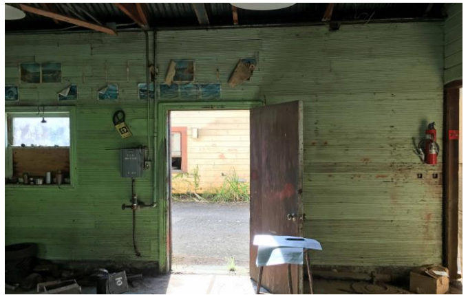
Figure 265 4.D door on the east wall to the roadway.
