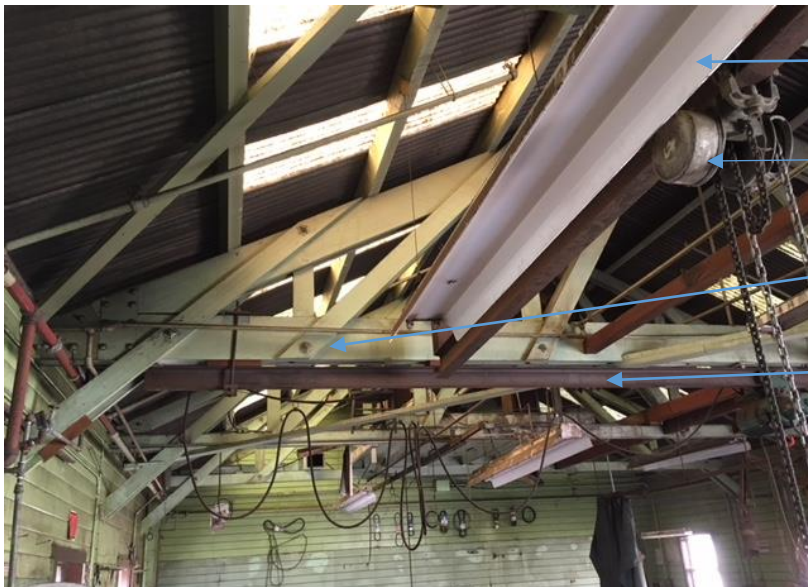
Figure 113 modified fan truss system and open ceiling.
