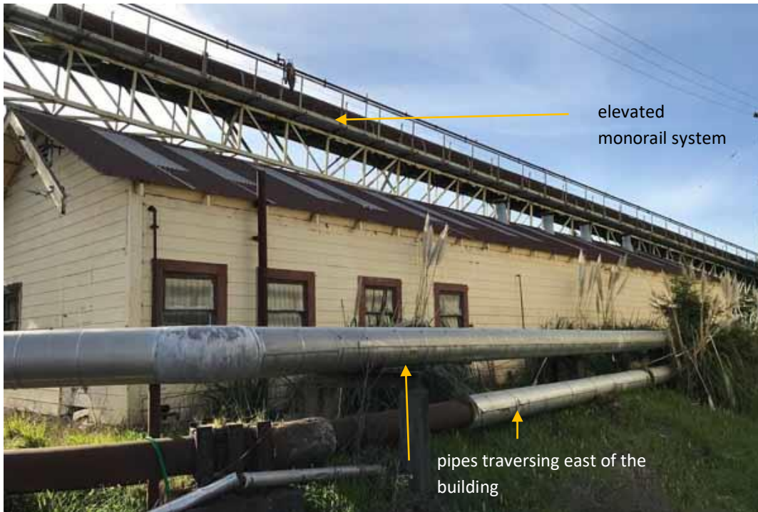
Figure 223 2.C monorail system running above to the west of the building, pipes along the east side of the building.
