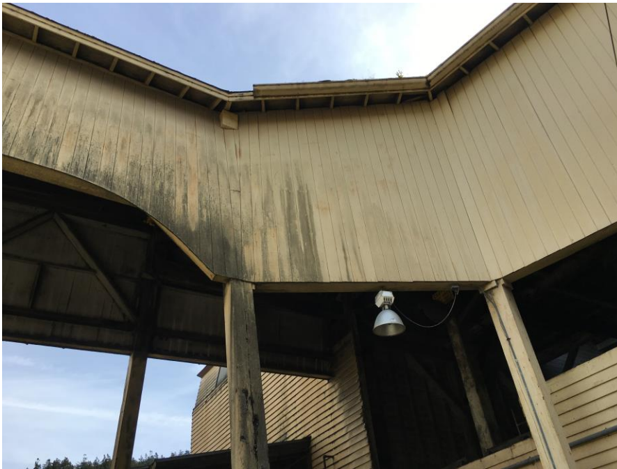
Figure 42 2.M exterior curved wall, open eaves, vertical wood sheathing, structural timber column, exterior lighting fixture.
