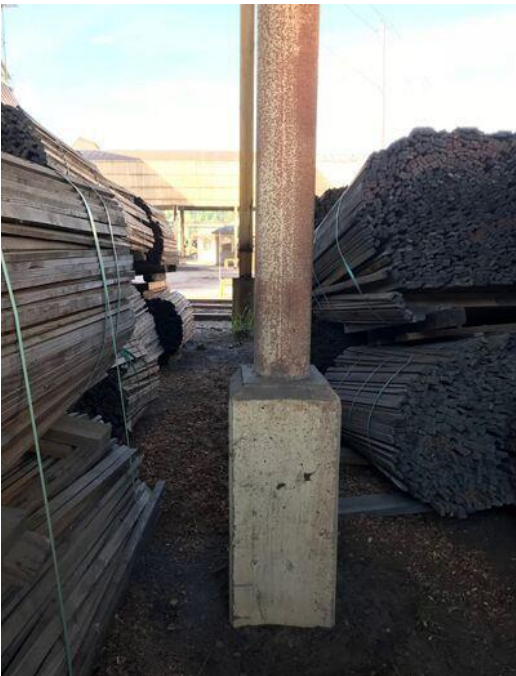
Figure 25 1.I typical 12 x 12 timber columns secured to reinforced concrete piers.
