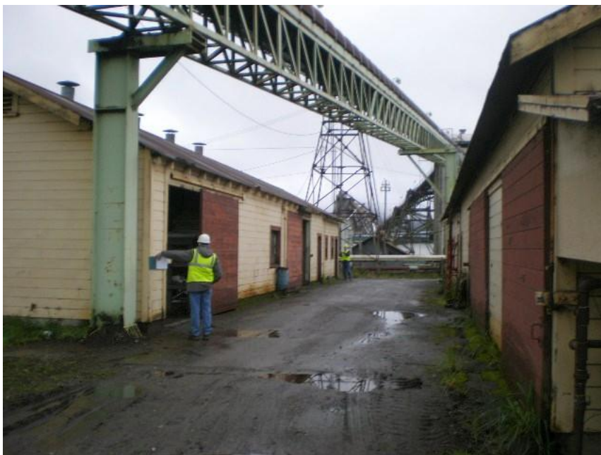
Figure 87 2.C east facing exterior wall from the north with monorail column.
