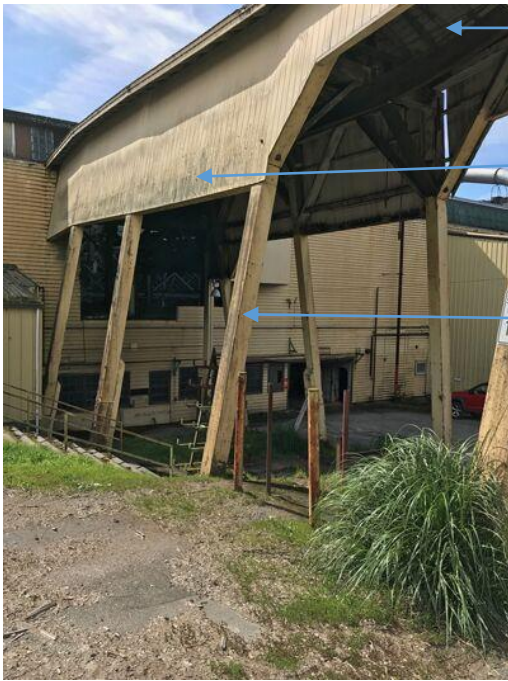
Figure 48 3.C wood siding, structure timber angled columns on north side of the tunnel.
