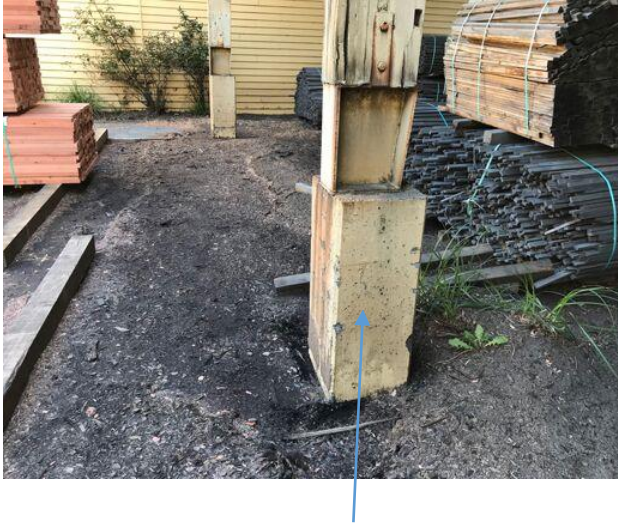
Timber column, foundation, metal straps, bolts.
