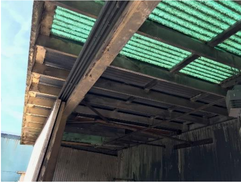
Figure 200 typical roof beams and translucent corrugated panels for light.
