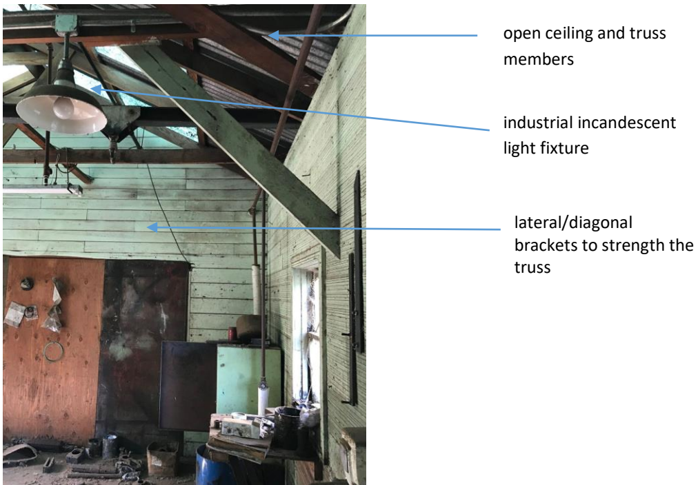
Figure 267 4.F lateral/diagonal brackets, open ceiling, truss, and industrial incandescent light fixture.
