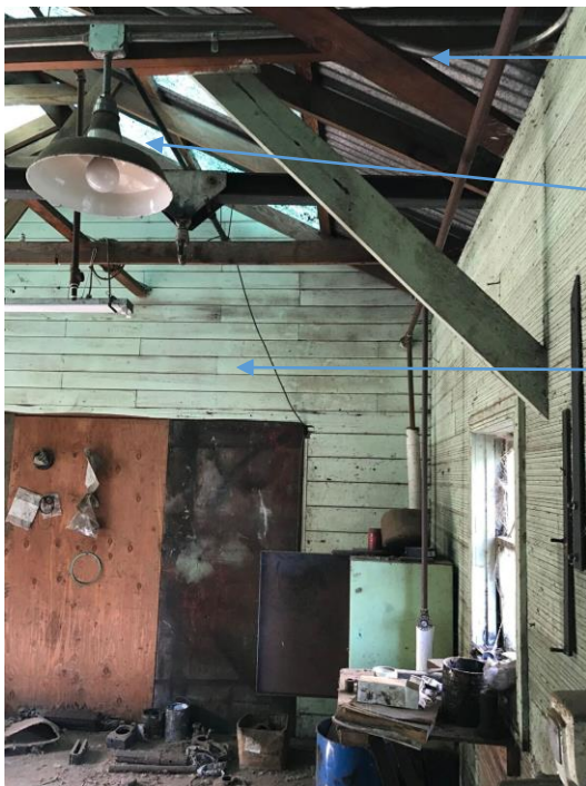
Figure 237 4.F lateral/diagonal brackets, open ceiling, truss, and industrial incandescent light fixture.
