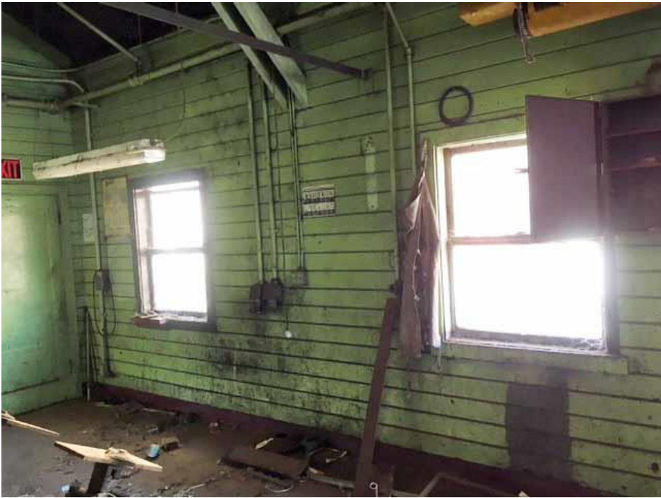
Figure 94 3.4 pair of double-hung wood windows with wood surround and frame, horizontal interior wood siding, electrical outlets.
