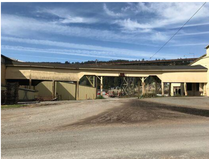
Figure 45 3.A Northern Monorail Tunnel view from the east.
