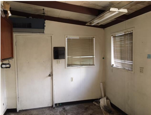
Figure 107 5.A addition, non-contributing.
