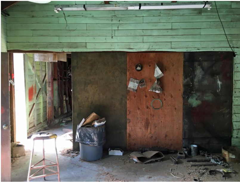
Figure 326 4.E opening and plywood boards used to reduce width of opening.
