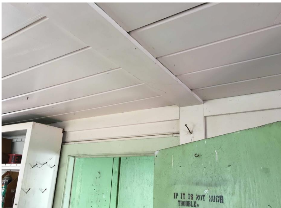
Figure 269 4.H wood planks used for ceiling of small office.
