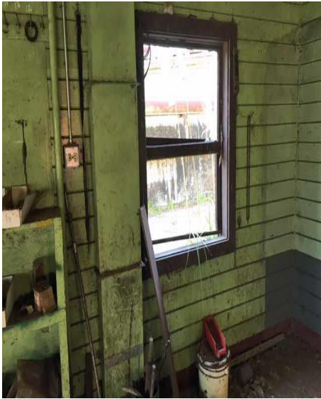
Figure 94 3.4 pair of double-hung wood windows with wood surround and frame, horizontal interior wood siding, electrical outlets.
