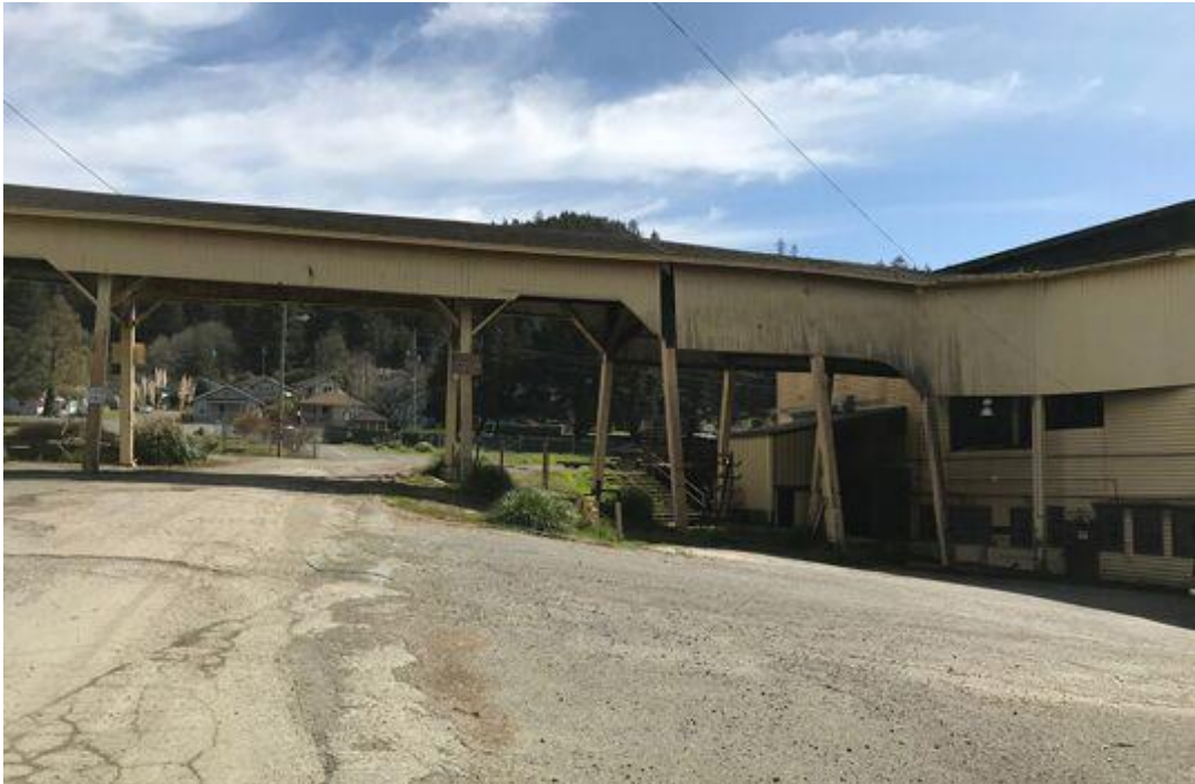
Figures 46, 47 3.B, 3C Northern Monorail Tunnel view from the west.
