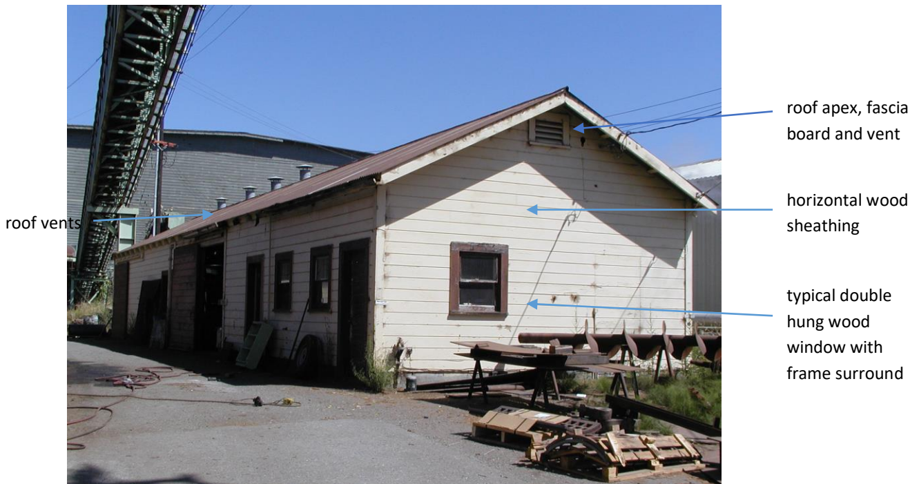
Figure 215 2.A south view of building, side-facing gable, typical double hung wood windows, wood doors, horizontal wood sheathing, vent at apex of north wall.
