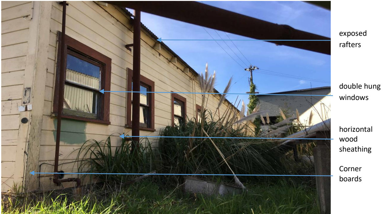
Figure 221 2.A east view of building, with double hung wood windows, frames and surrounds, horizontal wood sheathing, exposed rafters and corner boards.
