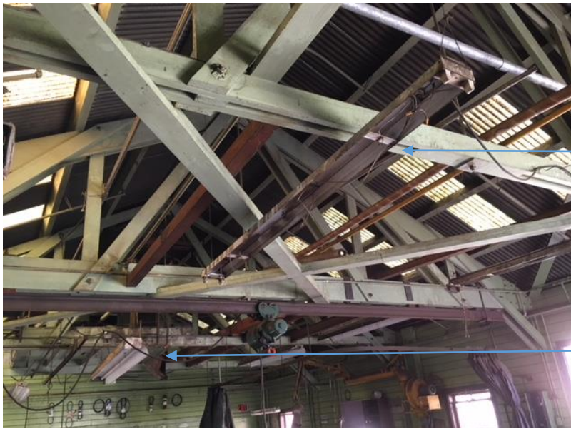
Figure 112 modified fan truss system and open ceiling.
