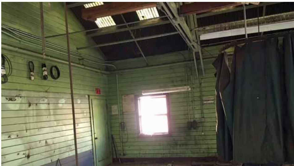
Figure 100 4.C partition wall, door, double hung wood window with frame and surround, lighting, open ceiling with translucent panels.
