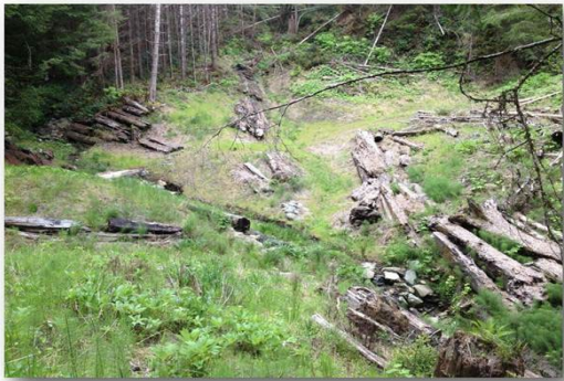
Decommissioned Road – Elk River Watershed
