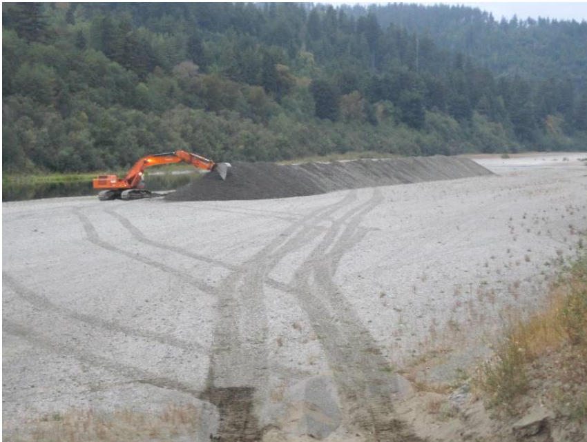
Figure 5. Excavator on Truck Shop Bar during 2012 operations (for example of operations).
