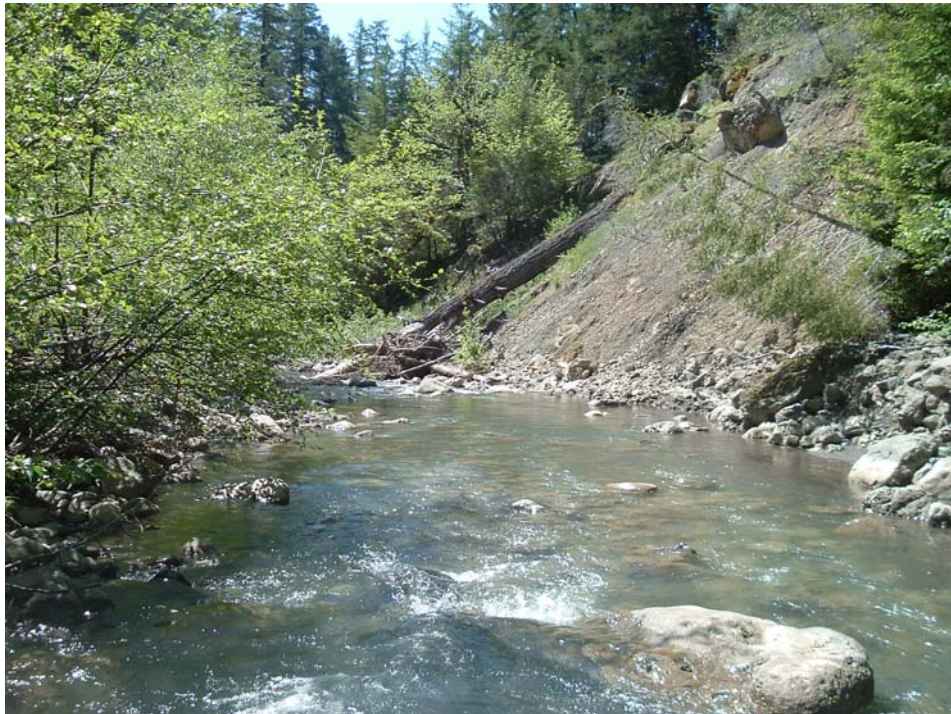
Photo 3-4. Rattlesnake Creek, streamside landslide, May 2005.
